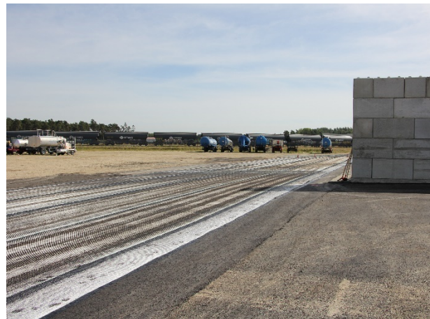
Figure 5: Test site fully covered with the asphalt reinforcement product
