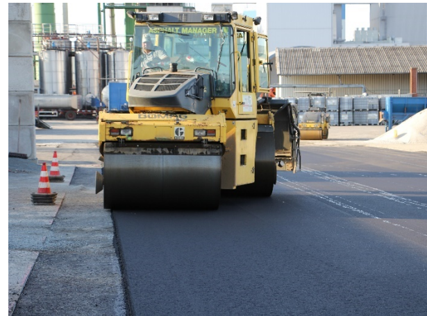
Figure 7: Installation of the top layer
