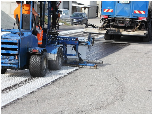
Figure 4: Installation of the asphalt reinforcement product using machinery
